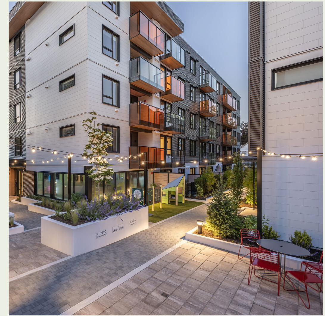
AT GROUND LEVEL, THE YARD FEATURES A TODDLER PLAY AREA, DOG RUN, AND THE PULSE FITNESS STUDIO.
